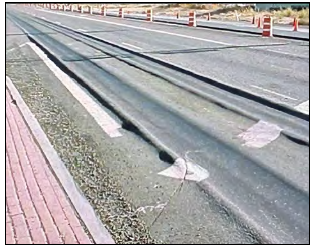
Note the cracks in the roadway
